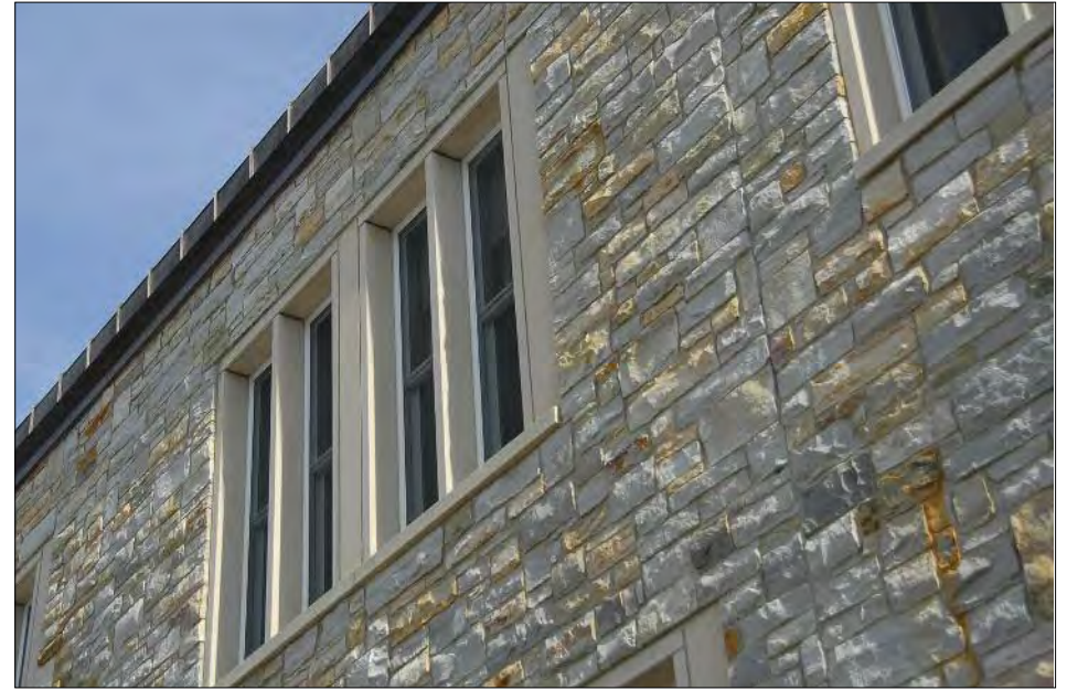
Above: Split-face blocks and Indiana Limestone masonry sills were chosen to complement the modern design of the Starr Axinn Center project amidst the traditional stone buildings of the Middlebury College campus. The "Middlebury College Blend" combined three local quarzitic sandstones.
